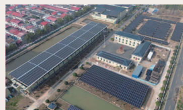
An Operational Water Plant in China
